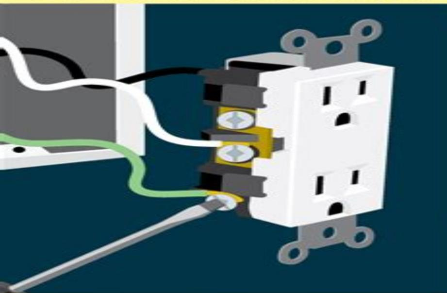
Using your flathead screwdriver tightly screw the wires into the new outlet.
